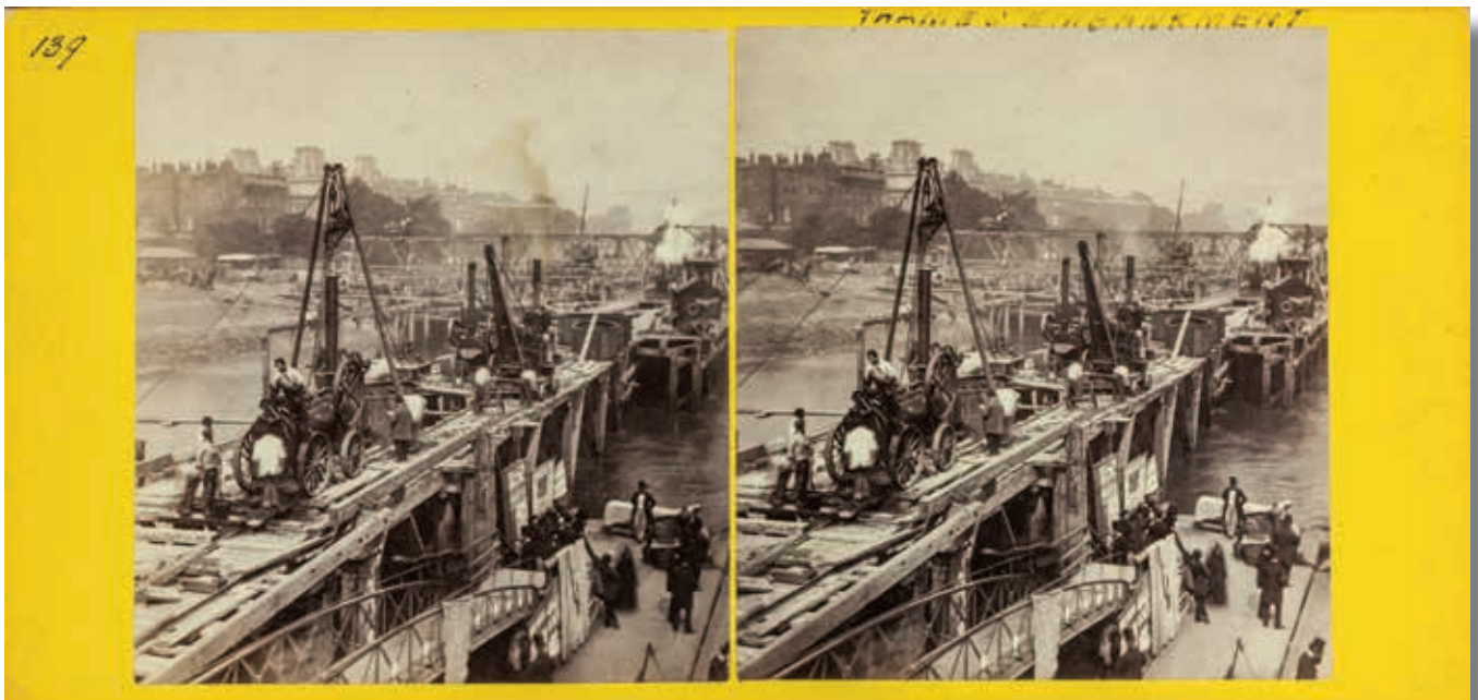
Building the Thames embankment c.1864, London, England
